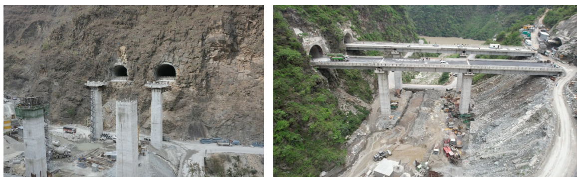
Figure 7. The steep natural slope at the western portal of tunnel T4-02.
