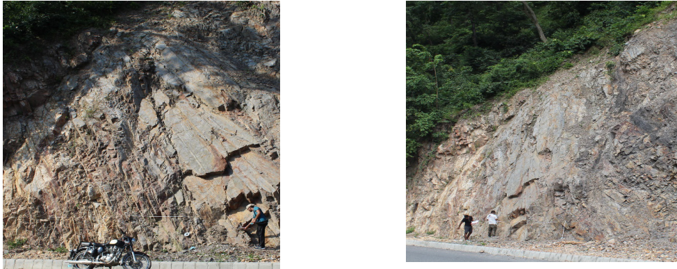
Figure 2. Scanline survey done on Slope 1.
