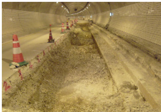
Re-investigation of original excavation surface under pavement concrete
