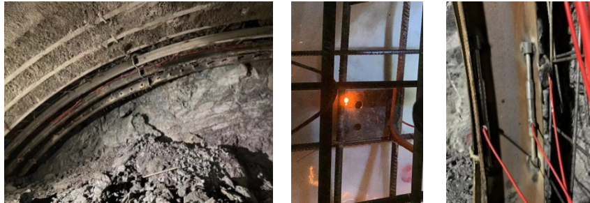
Figure 4. Installation and embedding of monitoring instruments.
