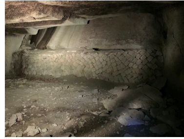
Figure 2. Internal view of abandoned underground quarry
