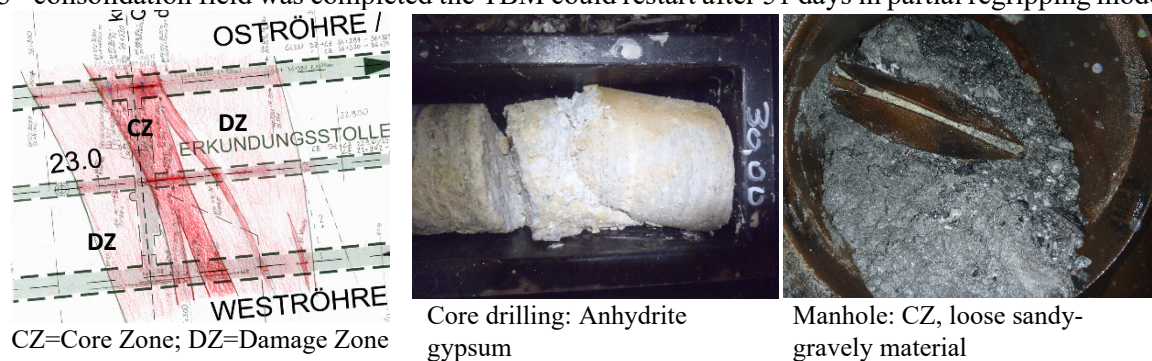
Figure 5. MT-W standstill at chainage 36+312. Model of the fault zone and photos of the fault material.
