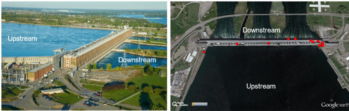
Figure 1. Left: Photograph of the Beauharnois Dam. Right: Plan view of the dam with approximate location of selected investigations boreholes (red dots).
