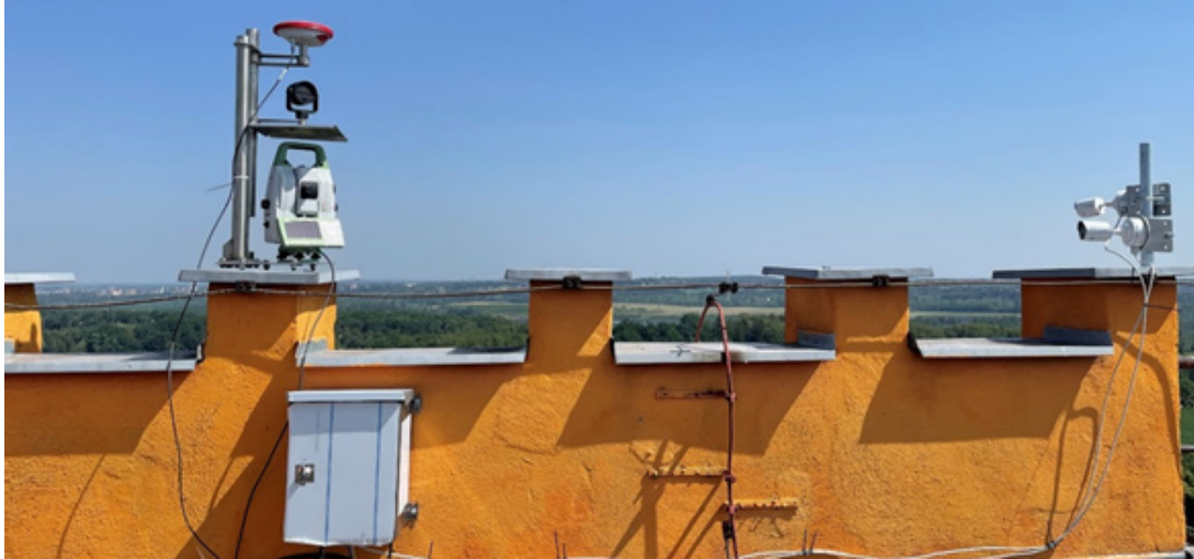
Figure 2. Monitoring set of Automatic Geodetic Monitoring System (CSM South).
