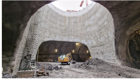
Figure 8. Central Access to Station during Construction.
