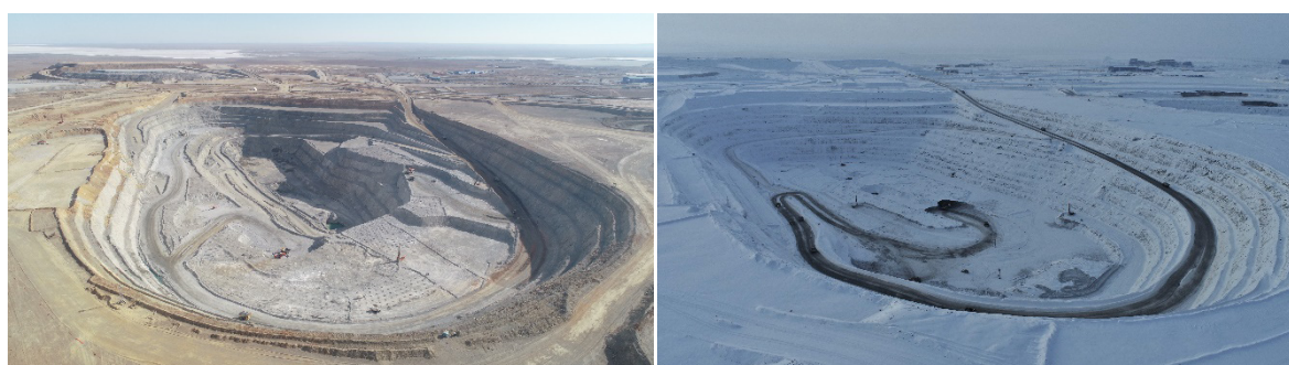
Figure 2. Aktogay Copper Mine Stage 2 Pushback: Looking South. Left: September 2021 (Autumn). Right: December 2022 (Winter).
