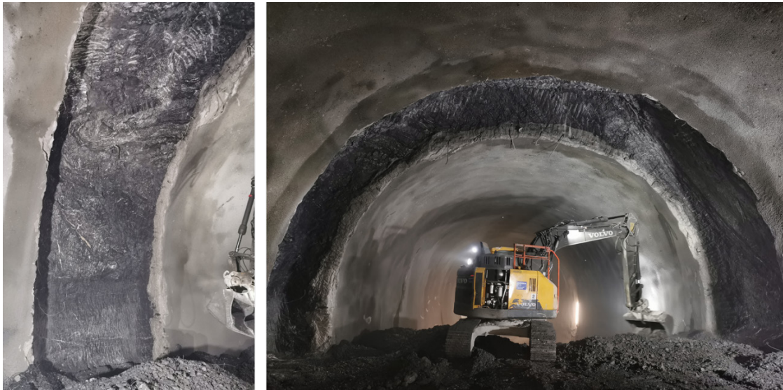
Figure 4. Photographs of the excavation of the shotcrete bulkheads.
