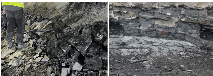
Figure 3. Blocky Slates with foliation dipping towards the excavation at North-wall.
