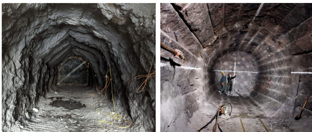
Figure 1. Example of tunnels with damage control system, to the left Drill & Blast of poor quality ( http://www.bradshawcc.com/projects/441/view/ ), to the right Drill & Blast of good quality (Kuzyl & Martino, 2008).
