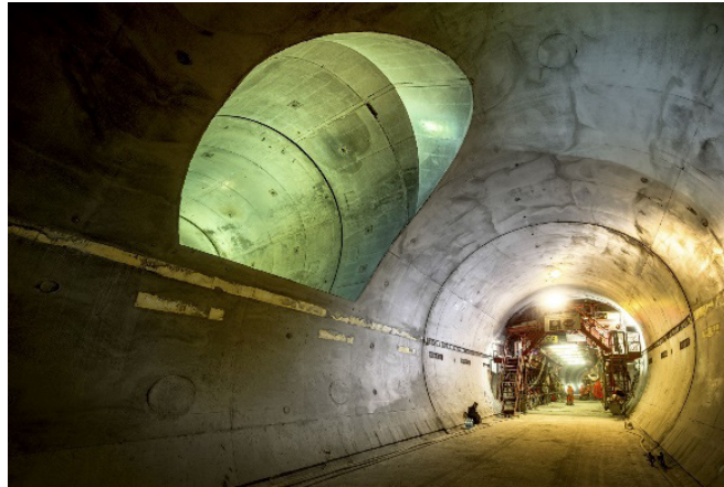
Figure 3. Concrete work for inner lining in emergency station. (ÖBB/Ebner).
