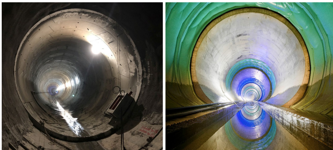
Figure 2. End of continuous driving and associated inner lining. (ÖBB/Wagner/Ebner).
