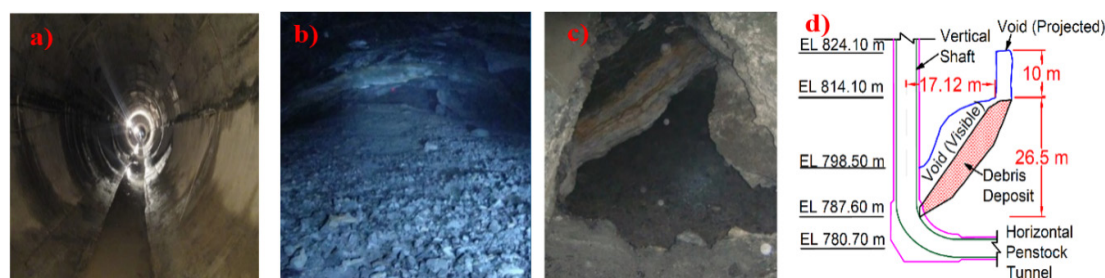
Figure 2. a) Vertical shaft; b) Large debris flow in vertical shaft; c) Cavity formation in the vertical shaft; d) Detail sketch of pressure shaft (Modified after Shah 2014).
