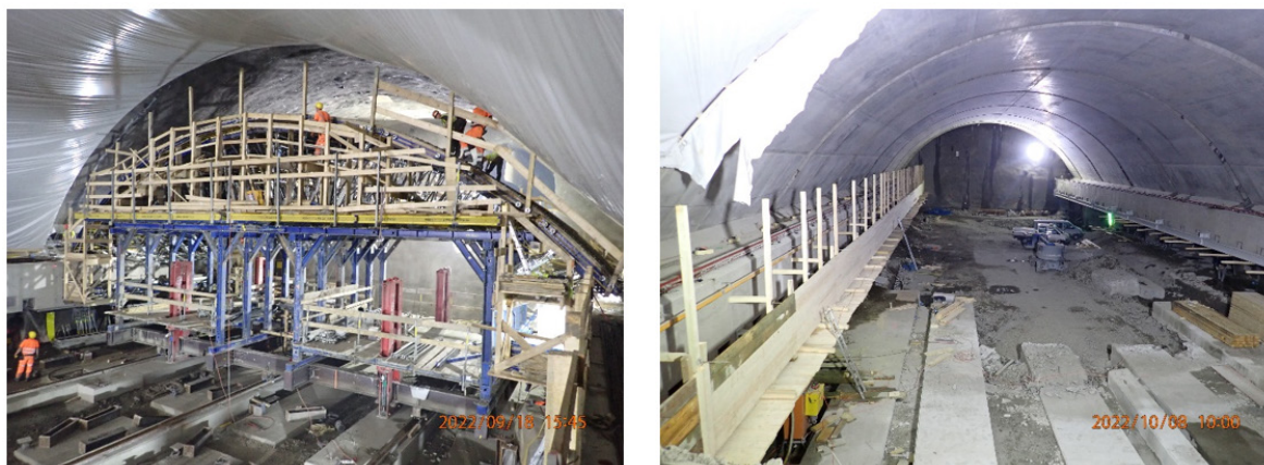
Figure 6. formwork carriage in low-position (left), finished inner lining (right).
