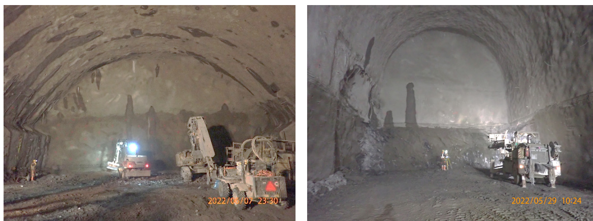
Figure 5. Status of Work machine cavern 07 May 2022 (left), transformer cavern 29 May 2022 (right).
