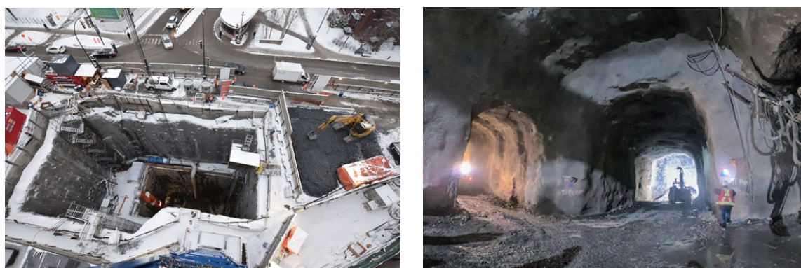
Figure 3. Excavation of EMP Station entrance shaft and tunnels.
