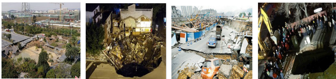
Figure 1. Cases of surface subsidence and collapse caused by tunnel construction.
