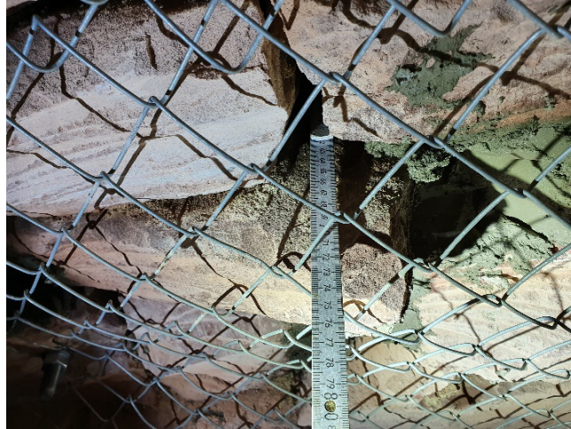
Figure 2. Loosened and temporarily secured sandstone block [source: Boley Geotechnik GmbH].
