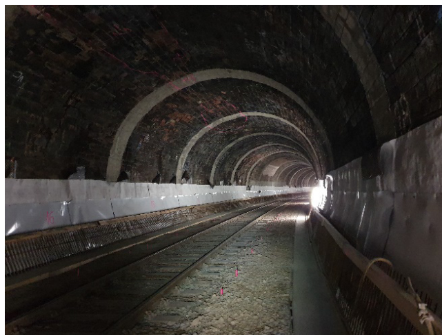
Figure 1. Existing shell of mortared sandstone blocks [source: Boley Geotechnik GmbH].
