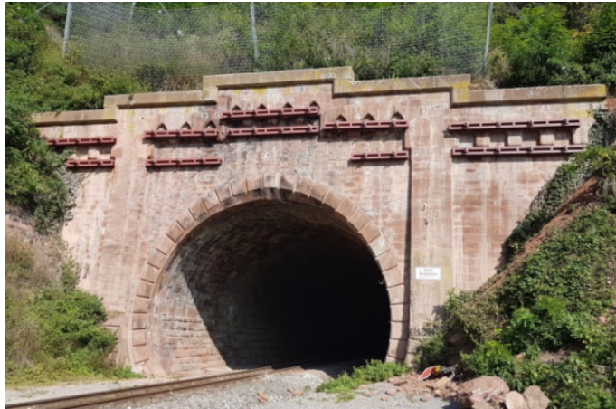
Figure 5. Tunnel portal with temporary retaining system [source: Boley Geotechnik GmbH].
