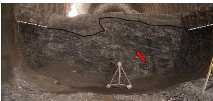
Figure 1. Face images of the bench/invert excavation with distinct failure mechanisms.
