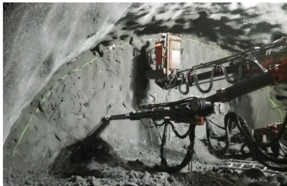
Figure 2. Top heading drilling operation with parallel drilling of two booms.
