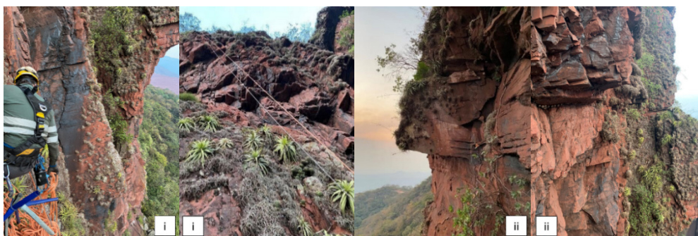
Figure 6. Typical condition of the rock face.
