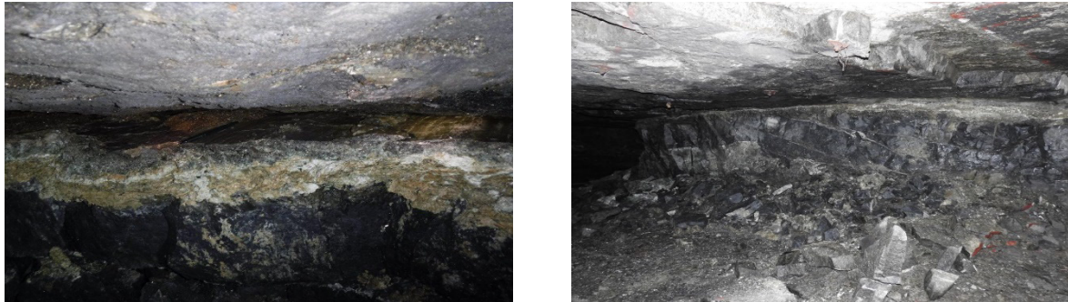
Figure 1. Underground photographs of the alteration layer present in the pillars at Everest Platinum Mine. Close up of the alteration layer (left). Pillar showing the presence of the alteration layer on the top contact of the chromitite pillar (right) (after Couto, 2022).
